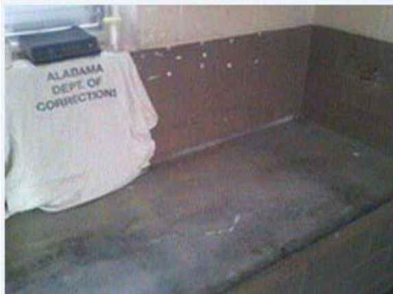
7c Concrete bed
